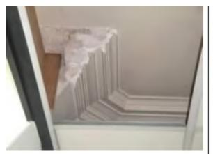
Typical cornice detail and damage incurred by alterations to windows/ installation of suspended ceilings.
